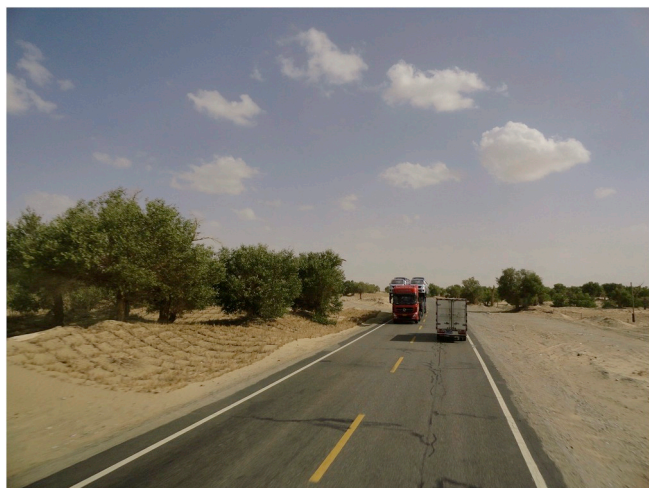
Fig. 6. Euphrates poplars together with reed grids stuck in the sand should keep the sand from encroaching onto the road. Photo: Author, 2011.
